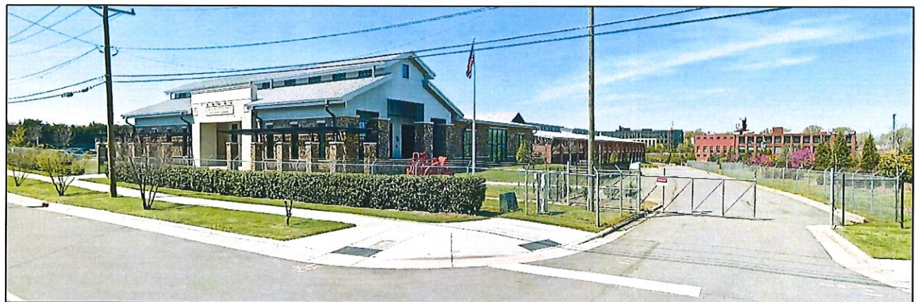
The rezoning site located along S. Clarkson Street (above and below).
